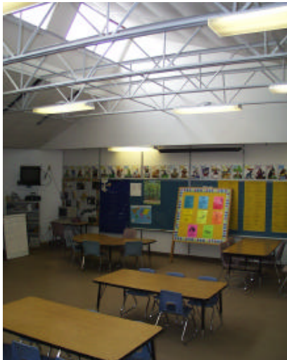
South Facing Monitor Skylights
