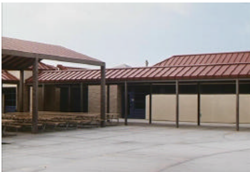
Type B Skylight School
