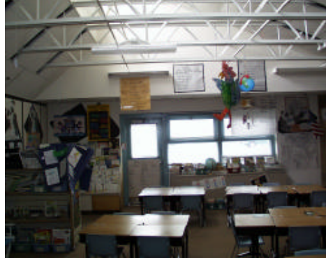
South Facing Monitor Skylights
