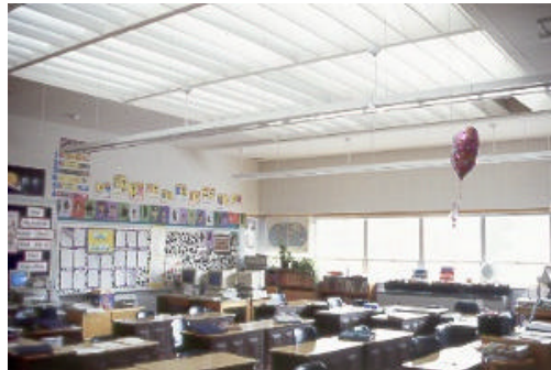
Central Skylight and Diffusing Louvers
